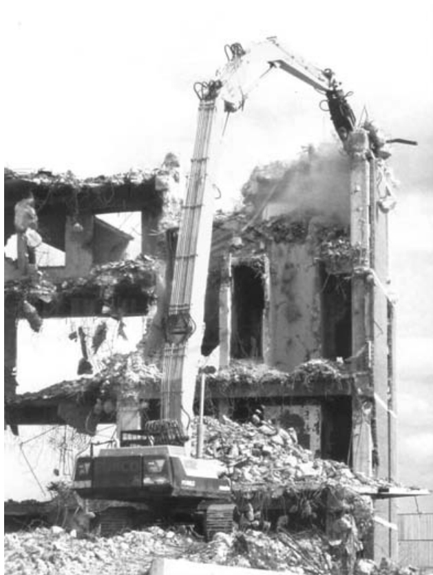
Figure 3: Crane-attached shear
